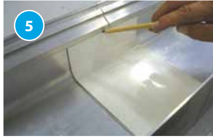
One edge of the joiner will require trimming down to allow it to clip into the groove on each side of the box gutter.
