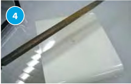
The plastic box gutter joiner can be found in the component box. File down the mould spur off the underside.
