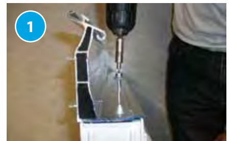
The Global eaves beam is designed to suit 60-70mm frames and is fitted using screw fittings. Fit the internal eaves beam face 2mm in from the inside frame line.
