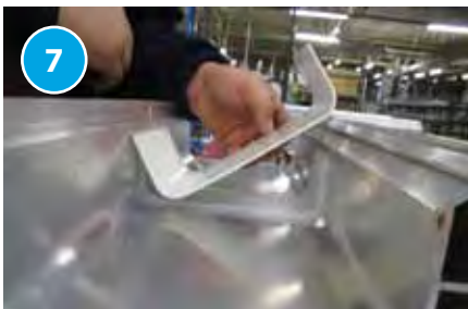
Clip the joiner into the back groove on the box gutter and rotate the joiner into position allowing it to clip into the front groove. Remove any excess sealant from each side of the joiner.
