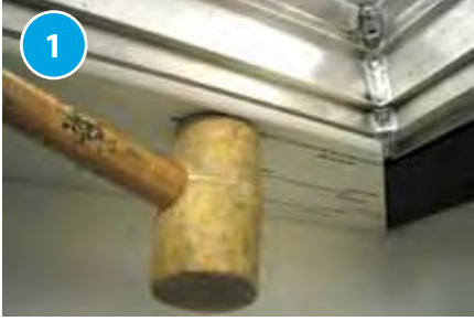
Box Gutter: Position then knock the box gutter under clad in to position using a rubber mallet.
