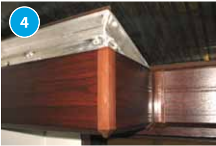
Raised Leg Box Gutter: Fit all of the internal side clads as standard.
