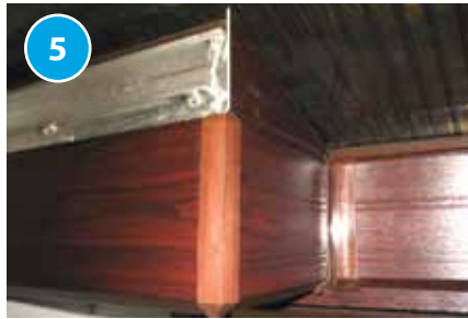
Extra box gutter under clad is supplied to cloak of the remaining raised leg section.
