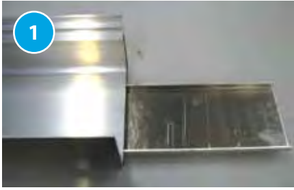
Slide the aluminium joiner half way into the body of one box gutter.
