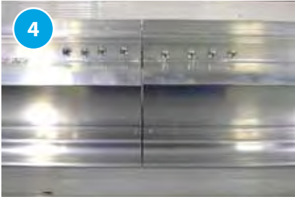
Slide the other ridge body onto the joiners and repeat the fixings procedure.
