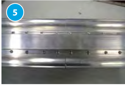
The view of the lower ridge joiner connected via 8 XM48-12 screws.
