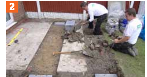
Construct the pads
