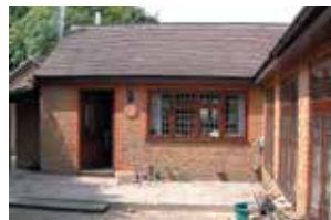
The existing site prior to conservatory installation
