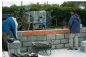
The concrete base and dwarf-walls are constructed
