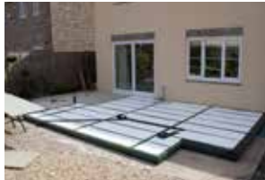
Insulation sheets fitted in to steel sections
