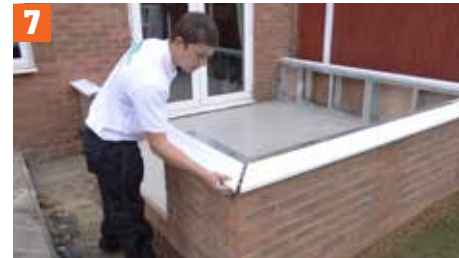
Install the conservatory
