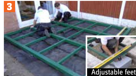
Bolt the sections together and to house wall
