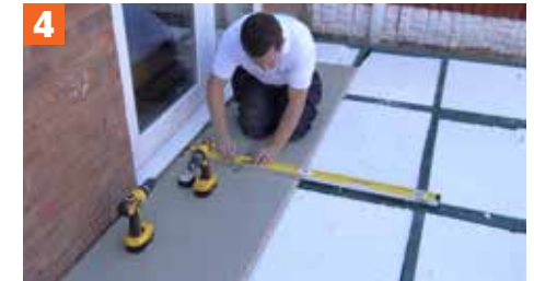
Fit the insulation and flooring
