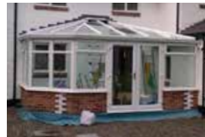
French doors are fitted
