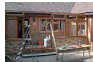
The PVCu frames are fitted into place
