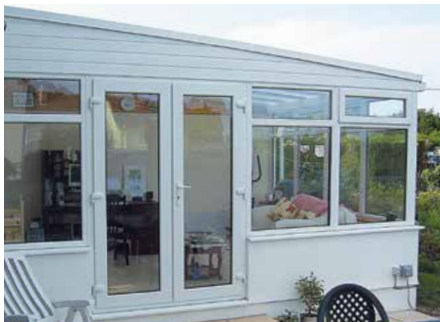
The conservatory is now complete and furnished for the perfect result
