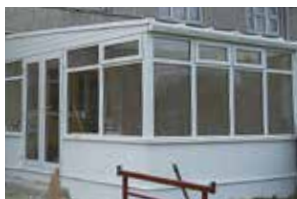
The external dwarf-walls are rendered and painted
