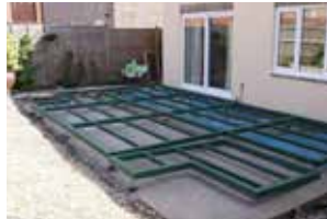
Steel sections bolted together and to house wall
