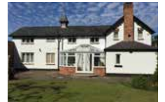
Conservatory is complete and ready to use
