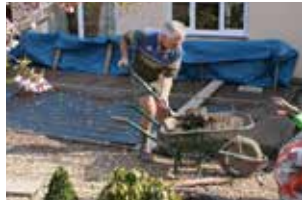
Site cleared & pads laid prior to ConservaBase installation
