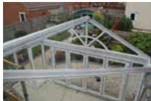
Conservatory frames and roof are installed
