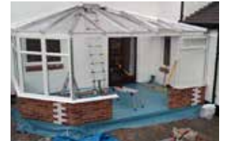
Modular steel walls, conservatory frames & roof installed
