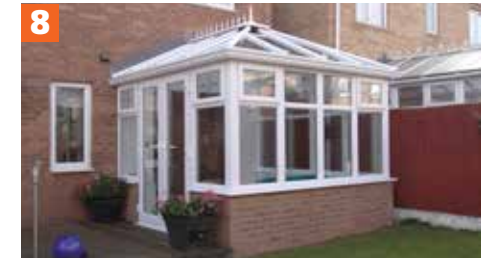
Indistinguishable from conventional build
