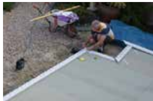
Timber floor fitted and conservatory cill positioned
