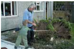
Site cleared prior to base and dwarf-walls being constructed
