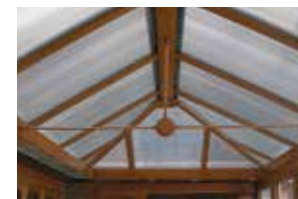
The tie-bars, roof glazing and PVCu cappings are fitted
