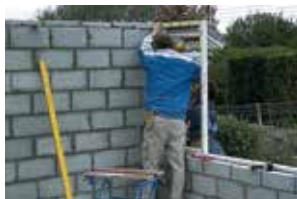
The PVCu external cill and frames are fitted into place
