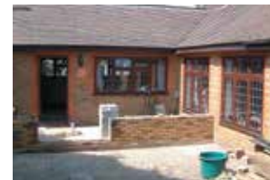
The concrete base and dwarf-walls are constructed
