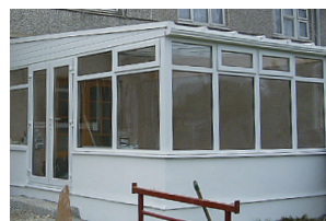
The external dwarf-walls are rendered and painted
