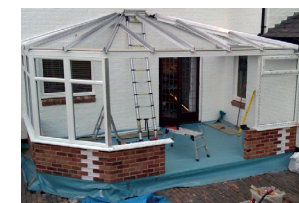
Modular steel walls, conservatory frames & roof installed
