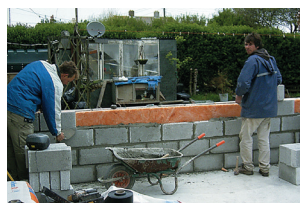
The concrete base and dwarf-walls are constructed
