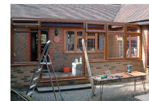
The PVCu frames are fitted into place
