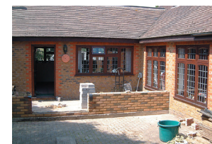
The concrete base and dwarf-walls are constructed
