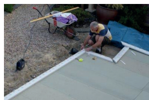
Timber floor fitted and conservatory cill positioned
