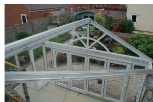
Conservatory frames and roof are installed
