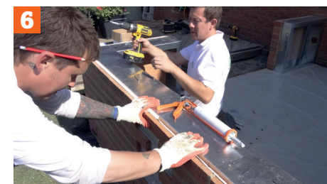
Secure the walls together and to the base
