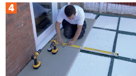
Fit the insulation and flooring
