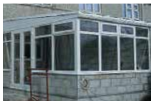
All glazing, PVCu cappings and PVCu cladding fitted
