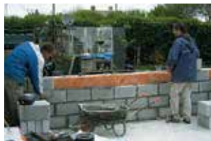
The concrete base and dwarf-walls are constructed
