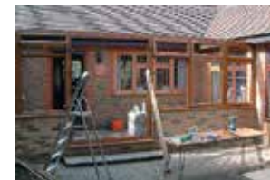
The PVCu frames are fitted into place
