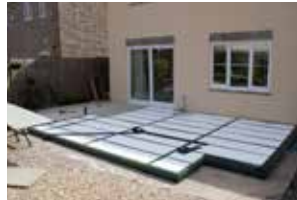
Insulation sheets fitted in to steel sections
