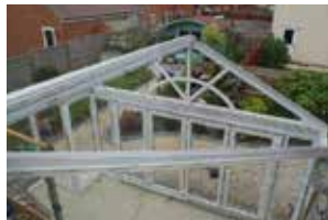
Conservatory frames and roof are installed
