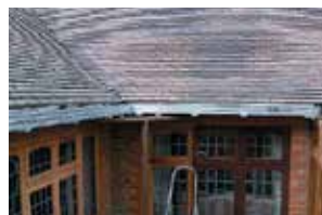
The aluminium ring beam and box gutters are fitted
