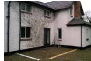
Site is marked out in accordance with the Pad Plan
