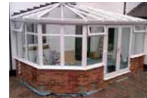
Extra brick slips (supplied) fitted to finish wall joints
