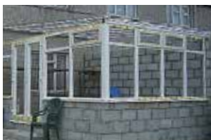
The aluminium roof wall-plate and rafters are fitted
