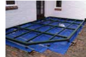
Pads are laid and steel sections bolted together
