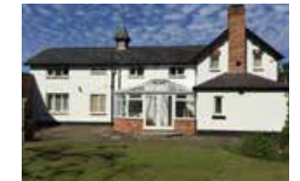
Conservatory is complete and ready to use
