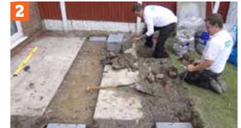
Construct the pads
