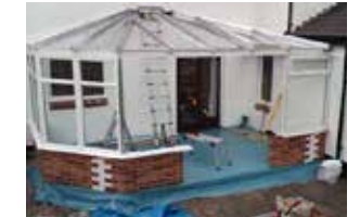
Modular steel walls, conservatory frames & roof installed
