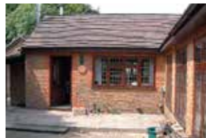
The existing site prior to conservatory installation
