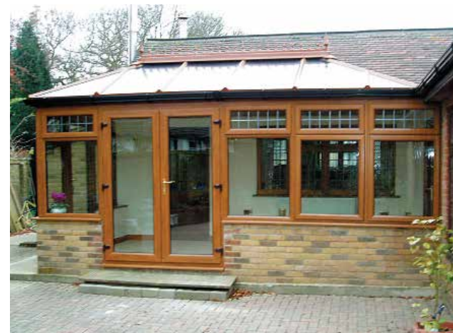
The double glazed units are fitted in the frames and this Hipped-Back Edwardian conservatory is now complete
