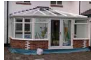
French doors are fitted
