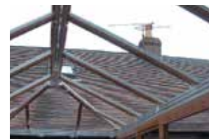
The aluminium ridge and roof rafters are fitted
