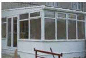
The external dwarf-walls are rendered and painted
