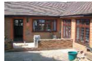
The concrete base and dwarf-walls are constructed
