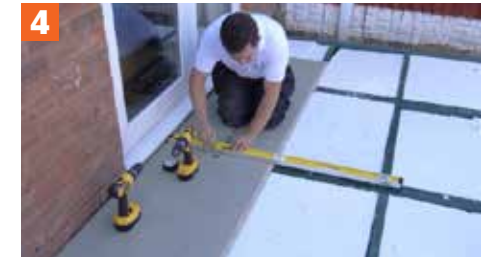
Fit the insulation and flooring
