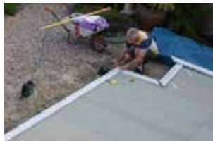
Timber floor fitted and conservatory cill positioned
