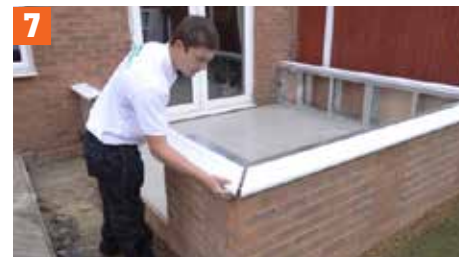
Install the conservatory
