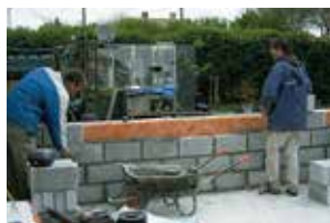
The concrete base and dwarf-walls are constructed
