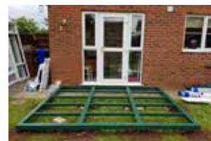
The steel ConservaBase is laid down quickly and easily
