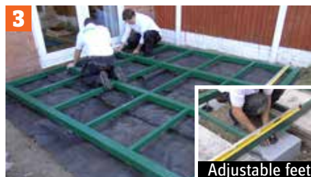
Bolt the sections together and to house wall
