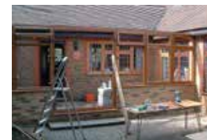
The PVCu frames are fitted into place
