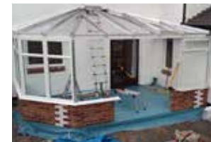
Modular steel walls, conservatory frames & roof installed
