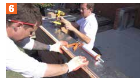
Secure the walls together and to the base
