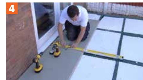
Fit the insulation and flooring
