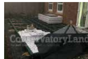
The ConservaBase lays the foundation for walls and frame
