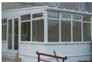
The external dwarf-walls are rendered and painted
