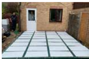
Once the ground is prepared, the ConservaBase is installed
