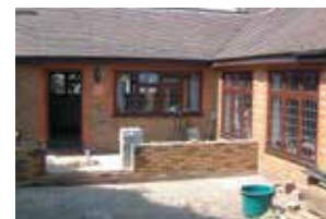
The concrete base and dwarf-walls are constructed
