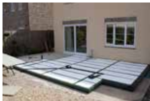
Insulation sheets fitted in to steel sections
