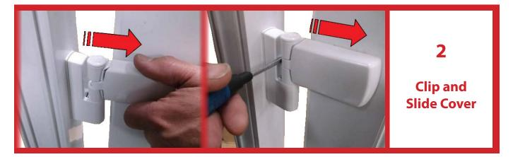
Pull the cover out towards the centre of the door. On release a click will be heard. If the cover does not open by hand, a scew driver can be used behind the knuckle to gently assist opening. Repeat stages 1 and 2.
