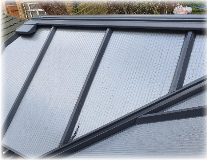
Valley Top Cap installed
