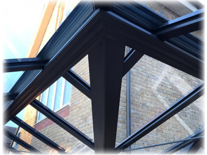
Valley Bottom Caps installed
