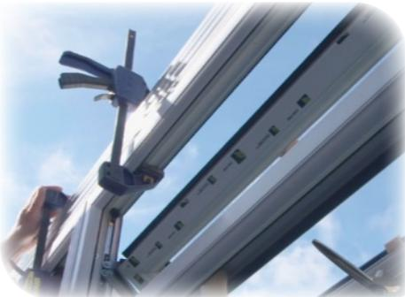
We recommend clamping your Ring Beam and frames before fixing the Ring Beam
