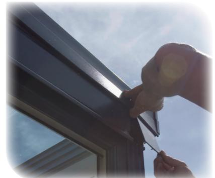
The Ring Beam End Cap will need to be trimmed to suit the pitch of your roof. Some standard pitches are marked on the inside for you as a guide. Glue / seal this to the end of the Ring Beam.
