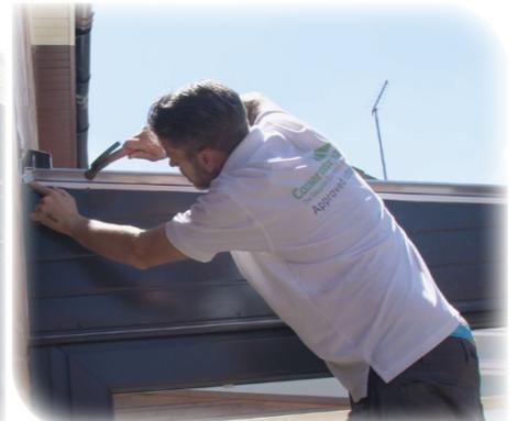
Draw a straight line between the points you have marked to give the cutting line for the first piece of cladding. Using a saw, cut the cladding to size. Offer this up and secure in place using a couple of the poly top pins supplied. Repeat this until you have completed both outside sections of the cladding.
