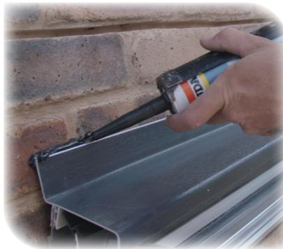
Next, run a bead of silicone along the top of the Wall Plate, or if your conservatory has a Low Line Wall Plate, silicone seal between the top of the aluminium Wall Plate and the property wall.
