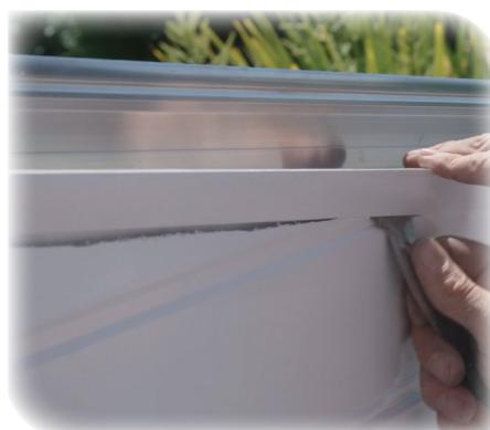
Complete the inner sections of cladding in the same way, but for the top exposed edge, cover this with the supplied Starter Trim as shown in the images on the left. This will require cutting to size, and you will need a sharp putty knife or similar to help when fitting the trim. Your Perlins are now complete.
