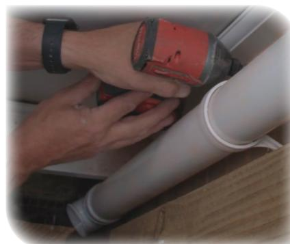
Fix the Downpipe Brackets to the wall. Four Downpipe Brackets are supplied with each Downpipe to use where required. Remember to fit the Shoe to the bottom of the pipe.
