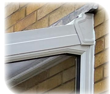
Glue / seal the Wall Plate end caps in place. Above left is an end cap for a standard Lean to Wall Plate, with an end cap for a Half Ridge Wall Plate shown above right. Please note, a Low Line Wall Plate is covered by the End Rafter Side Cap.
