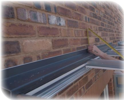
Start by measuring the height of the lead flashing required.
