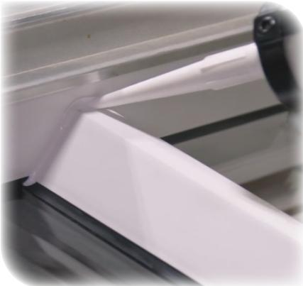
You must seal the Rafter Top Cap to the Wall Plate as shown above.
