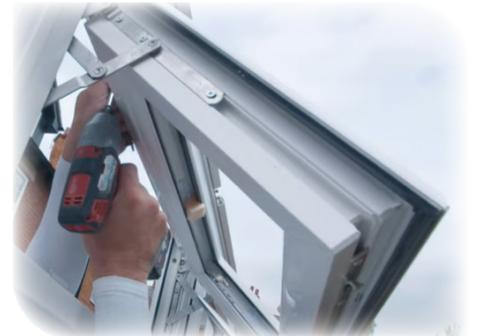
If you have opening windows, make sure the windows are open before fixing up into the Ring Beam
