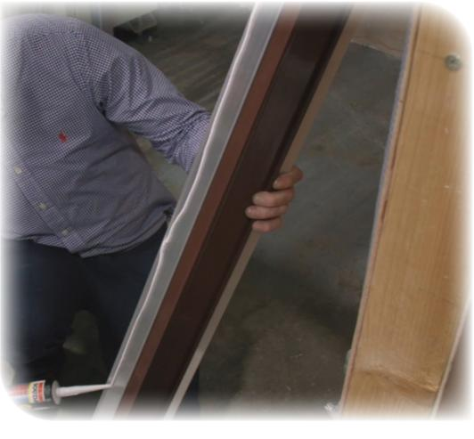
Before fixing the Ring Beam in place run a bead of silicone along the back edge of the ring beam. (You can test fit the Ring Beam to check its position first if required).
