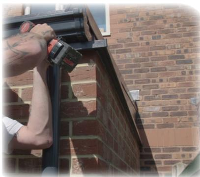
If you are running the Downpipe straight down from the Gutter, fit the Shoe to the bottom of the pipe, then fit the downpipe to the Universal Downpipe Adaptor (Spigot).
