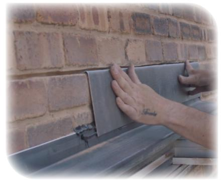
Now fit the lead into the ground out mortar line, and down over the top cap, or the aluminium Wall Plate depending on the type of Wall Plate you have. Refer to the image on the previous page.
