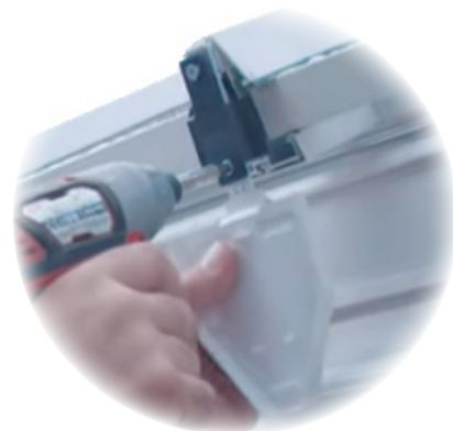
Fit a Rafter End Cap and Glazing Stop to the Rafter. For the End Rafters, you will notice the end caps are a different shape. The flat edge of the end cap sits to the outside on each side of the conservatory. Pull the glazing sheet back until it sits against the glazing end stops. Once in position peel away the yellow protective tape and gently pat the glazing down onto the Ring Beam seal adhesive tape.
