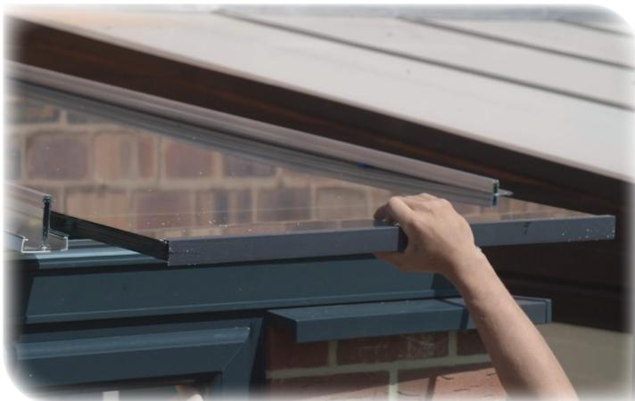
Slide the glazing panel on to the Rafters and into the Wall Plate glazing trim (remember to remove the protective film if your glazing is polycarbonate).
