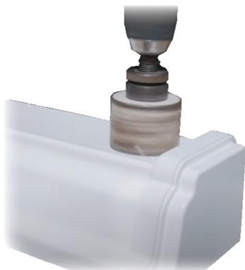
To fit the Spigot, first determine where the Universal Downpipe Adaptor is to go, and then drill a 53mm diameter hole in the Gutter using a hole saw.
