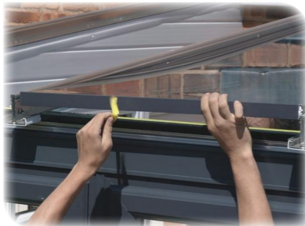
Pull back a small amount of the yellow protective tape back and fold it over. Do not remove it all at this stage.
