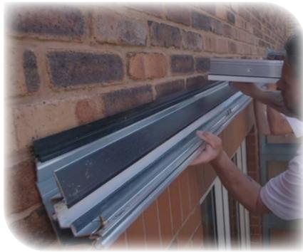
Now lift the Wall Plate to allow the rafters to fit to it, loosely tighten the bolts. The variable support that the rafters fix to will pivot forward to allow you to get the Wall Plate to the correct height. See your roof plan for this dimension. To find this dimension, please see the example roof plan on page 4 of this instruction.
