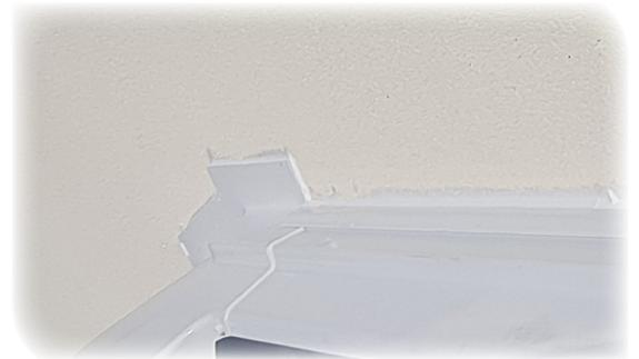
Next fit the assembled Top Cap and Radius Ends. Before you position the top cap in place apply a mastic / silicone seal to the areas of the Half Ridge End top cap that will butt up to the property wall. Secure the wall plate in position and complete the lead flashing,
