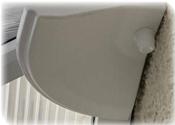
Once the Radius End bottom cap has been prepped (if required) secure it to the Nylon Threaded Bar, and add the decorative M10 boss to complete the internal finish. Simply screw in place.
