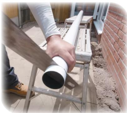
Measure the length of Downpipe required and cut to size. Take into account the Shoe, that fits to the bottom of the pipe, and any Offset Bends if you are using them.
