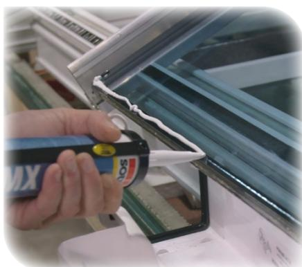
For self cleaning glass units only a specialised SMX sealant can be used. Run a bead of sealant along the top of the glass unit.
