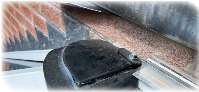
Fit the Foam Bung(s) over the top of the threaded bar and tighten the bolt in place at the top of the threaded bar as shown in the photo on the left. Once the Radius End Bottom Cap is in place, and the bolt on the underside tightened, it will pull the foam bung down tight to the glazing.
