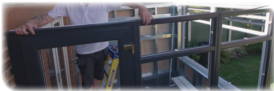
Before starting to construct your timber frame, you will need to fit the PVC Butt Joint and Head Drip to the top of the window / door frames. The PVC Butt Joints fits to the inside of the frame, and the Head Drip to the outer edge of the frames.
