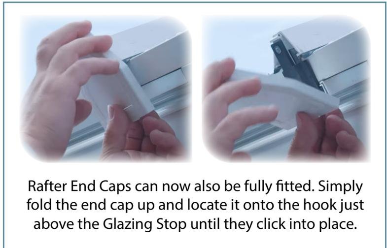
Rafter End Caps can now also be fully fitted. Simply fold the end cap up and locate it onto the hook just above the Glazing Stop until they click into place.
