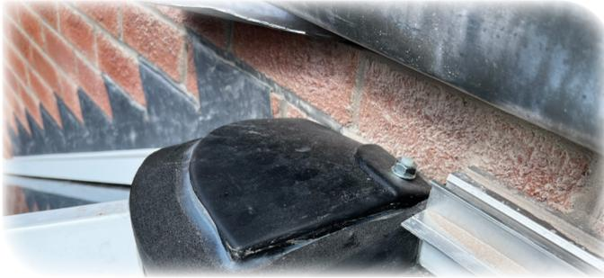
Fit the Foam Bung(s) over the top of the threaded bar and tighten the bolt in place at the top of the threaded bar as shown in the photo on the left. Once the Radius End Bottom Cap is in place, and the bolt on the underside tightened, it will pull the foam bung down tight to the glazing.
