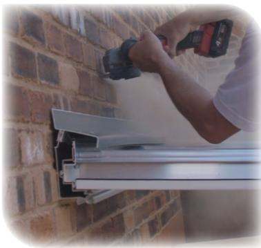
Next, using an angle grinder, grind out the mortar line ready to install the lead flashing
