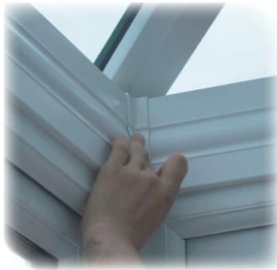
Most Lean-to conservatories only have a Ring Beam across the front. Ring Beam corner trims are only applicable to Hipped Lean-to's or Lean to's with a Ring Beam on the side.
