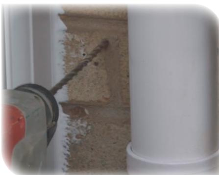
If you are attaching the Downpipe to your property wall you will need to pre drill any fixings that you choose to use, before fixing the Downpipe Brackets.
