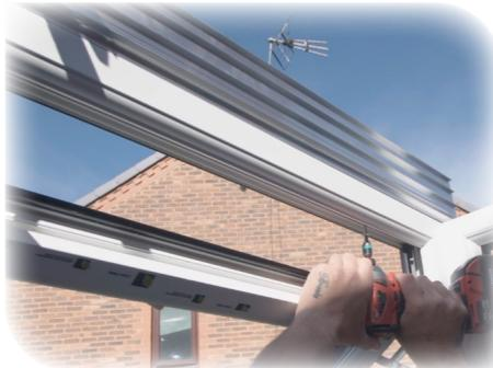
Using the 70mm self drilling fixings, fix up through the frame into the Ring Beam. Use 2 per frame or 2 per door sash
