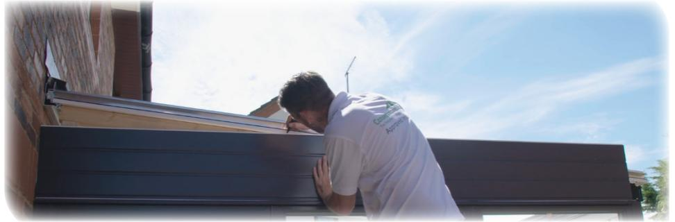
You will need the supplied Hollow Clad to finish off the Perlins. Offer up a length to the timber frame and carefully mark the top and bottom points that need cutting. The side cladding for the end rafters will cover the cuts at the top, but try and mark and cut the cladding as neatly as possible.
