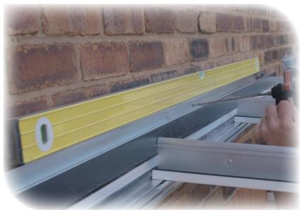
Ensure the Wall Plate is level both vertically and horizontally before drilling through the whole Wall Plate with a 6mm pilot hole, then fix in place using the 100mm direct to brick fixings. Add the remaining rafters and fully tighten all the bolts on the rafters.
