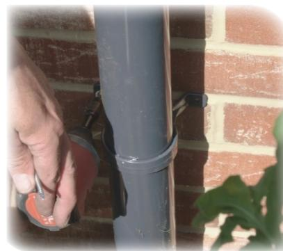
Fit the Downpipe Brackets to the wall or corner post for example, and the Downpipe installation is complete for this down pipe configuration.
