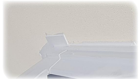
Next fit the assembled Top Cap and Radius Ends. Before you position the top cap in place apply a mastic / silicone seal to the areas of the Half Ridge End top cap that will butt up to the property wall. Secure the wall plate in position and complete the lead flashing,
