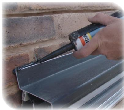
Next, run a bead of silicone along the top of the Wall Plate, or if your conservatory has a Low Line Wall Plate, silicone seal between the top of the aluminium Wall Plate and the property wall.
