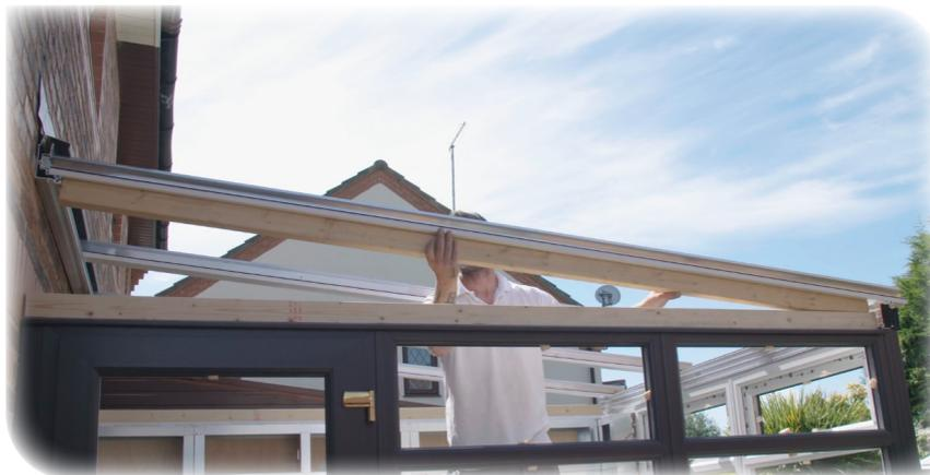
Start by constructing your timber frame. Use 50mm wide timber. The timber should be central to the rafter leaving a 10mm gap each side for the PVC Hollow Clad. You can secure the timber in place by fixing down through the end roof rafters, and up through the conservatory frames.
