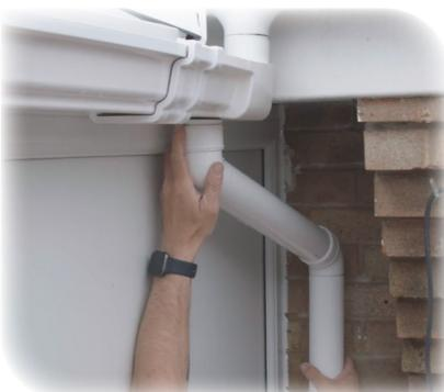
If the Downpipe is to be positioned away from the Gutter you may need to use the 112° Offset Bends and your offcut of Downpipe as shown in the example above.
