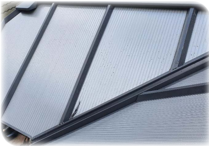
Valley Top Cap installed
